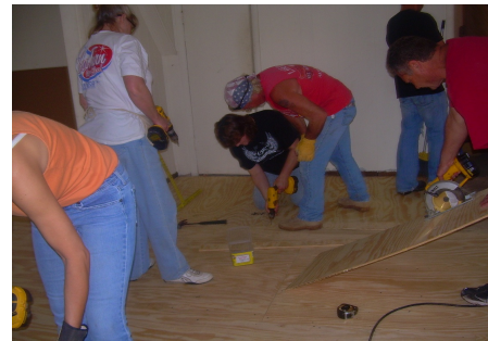
Westmoore crew working at the OKC Compassion transition house
